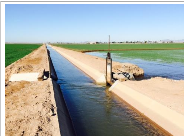
Figure 3.6a Concrete Lined Ditch
