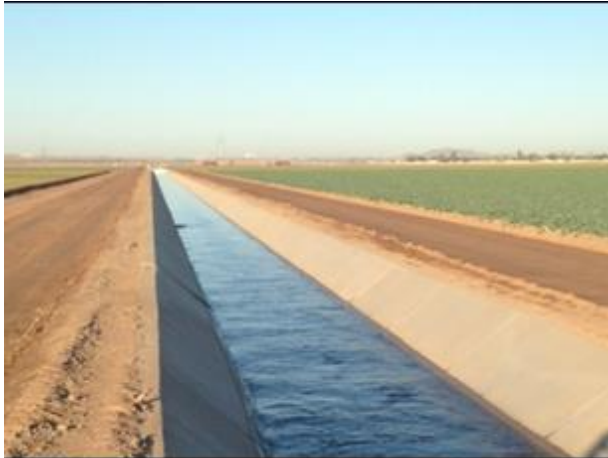
Figure 2.1 Concrete Lined Canal
